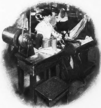
EXAMINING THE FABRICS FOR DEFECTS.
